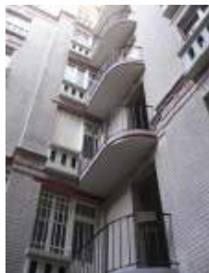
Renforcement coursives façade cour
